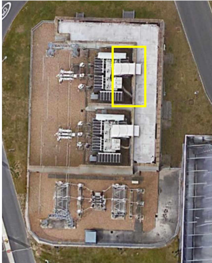
Figure 4 - Aerial View of R1 Step-up Transformers (Approximate Location of Figure 5 Below Boxed in Yellow)
